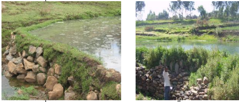
Figure 3. Diversion structure in Beles Traditional irrigation scheme
