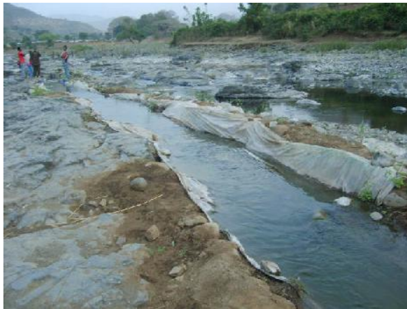
Figure 5. Diversion structure and primary canal at Zarima
