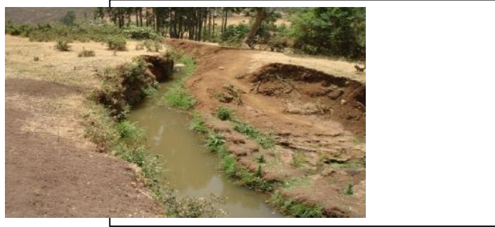
Figure 14. Unstable ditches
